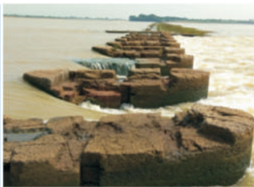
Fig. 32. Naraj barrage upstream
